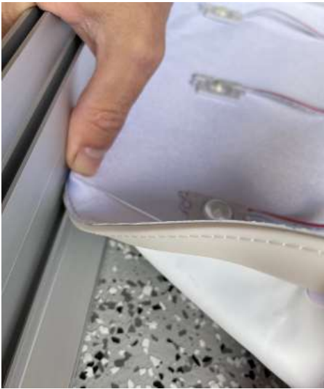
Gasket Installed in third opening
