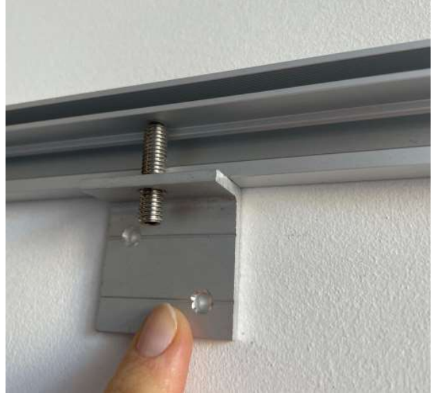
Wall Bracket @ top of frame
